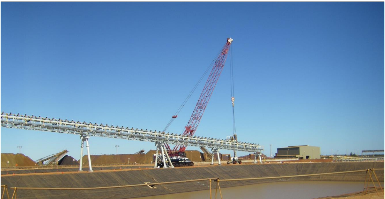
Figure 3: Utah Point Yard 2 conveyor installation works underway
