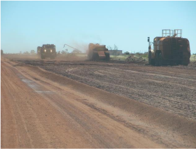
Figure 2: Abydos Mine haul road development works
